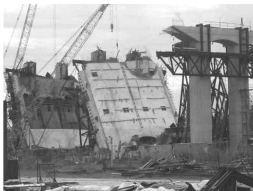
**Figure 1.** Bridge collapse during construction stage<sup>2</sup>.
