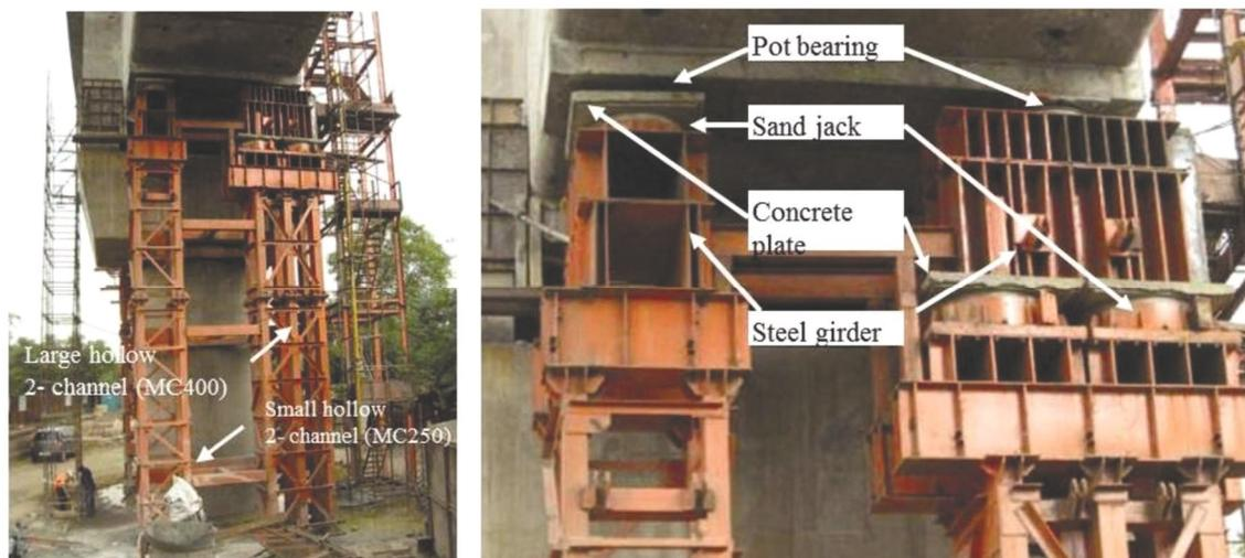
Figure 12. Details of temporary steel trestles.
