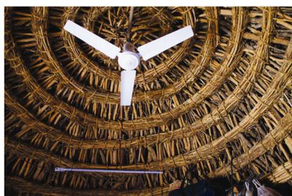
Fan and tube light inside the home deployed with inverterless system.
